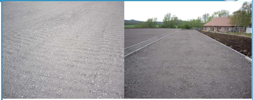
Finished sub-base layer paved to final tolerance
